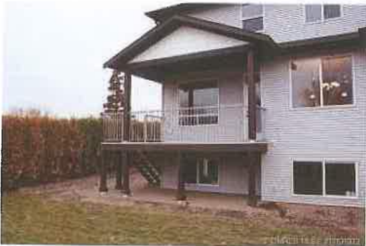
Basement partially out of the ground.
